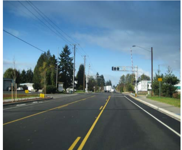
NE 88 th Street – completed October, 2009
